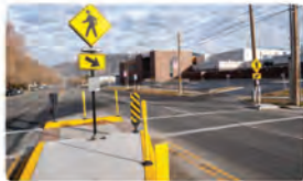
Flashing Crossing Beacons
